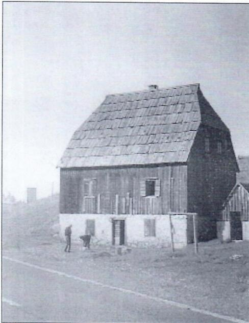
"Durmitorska" house is stone upon the ground and wood upon the stone. With a batten roof and cut gable (or triangular shape), it alludes to austere forms.
